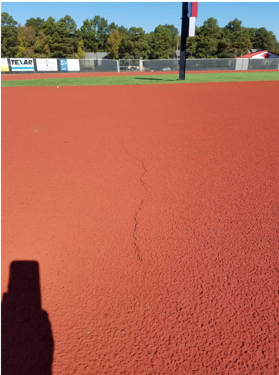
Example of a surface crack.
