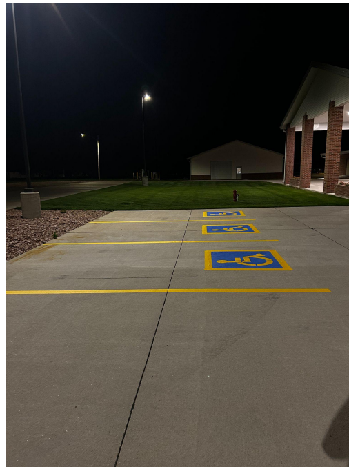
ADA Handicap Stalls with Access Aisles
