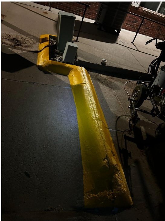
Curb Painting Detail — Night
